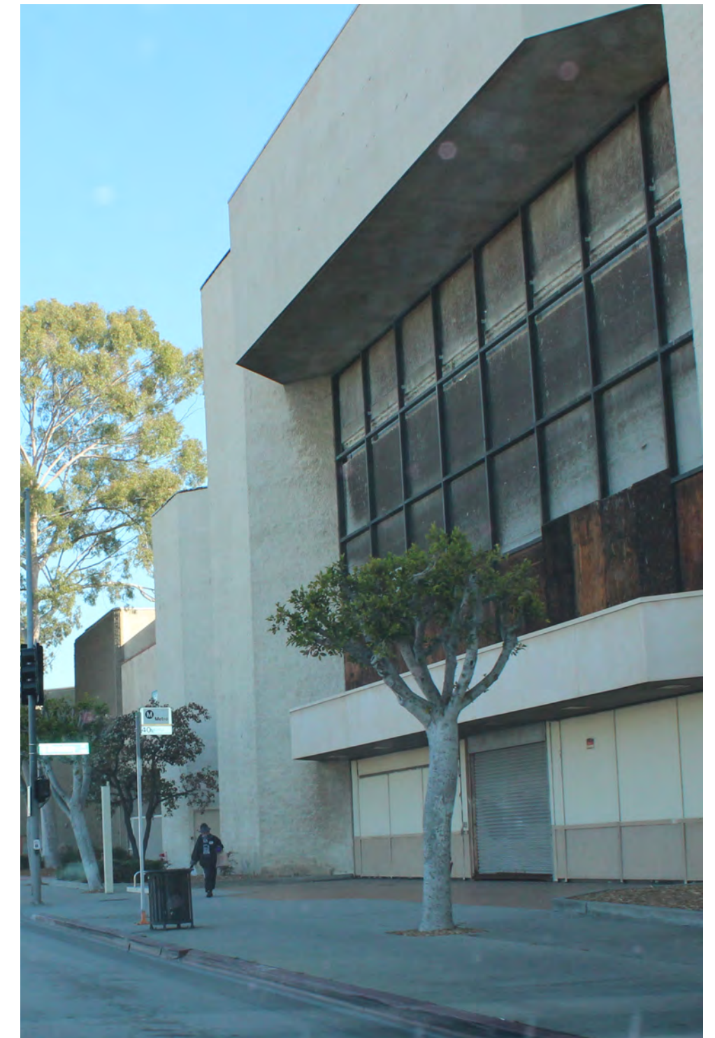
The Hawthorne Mall site presents an opportunity to create catalytic retail or mixed-use development on Hawthorne Boulevard
