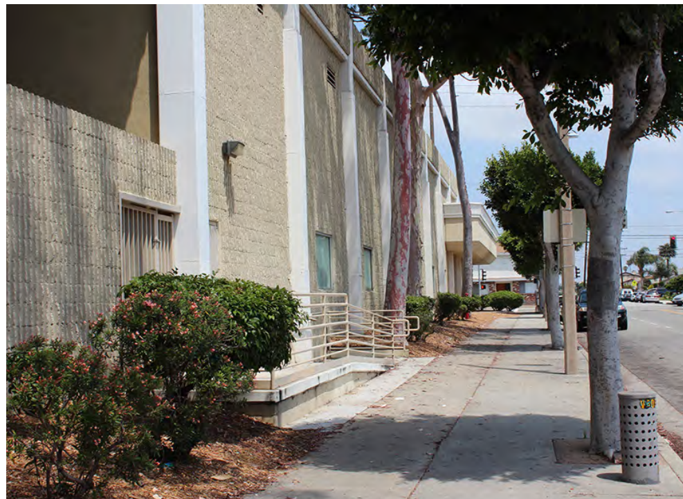
Hawthorne Mall's street frontage needs improvements
