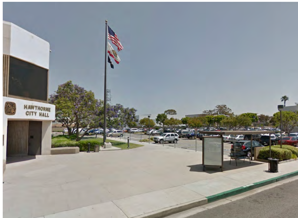
City Hall has some open space and elements of a public plaza that should be improved and expanded as part of a comprehensive design
