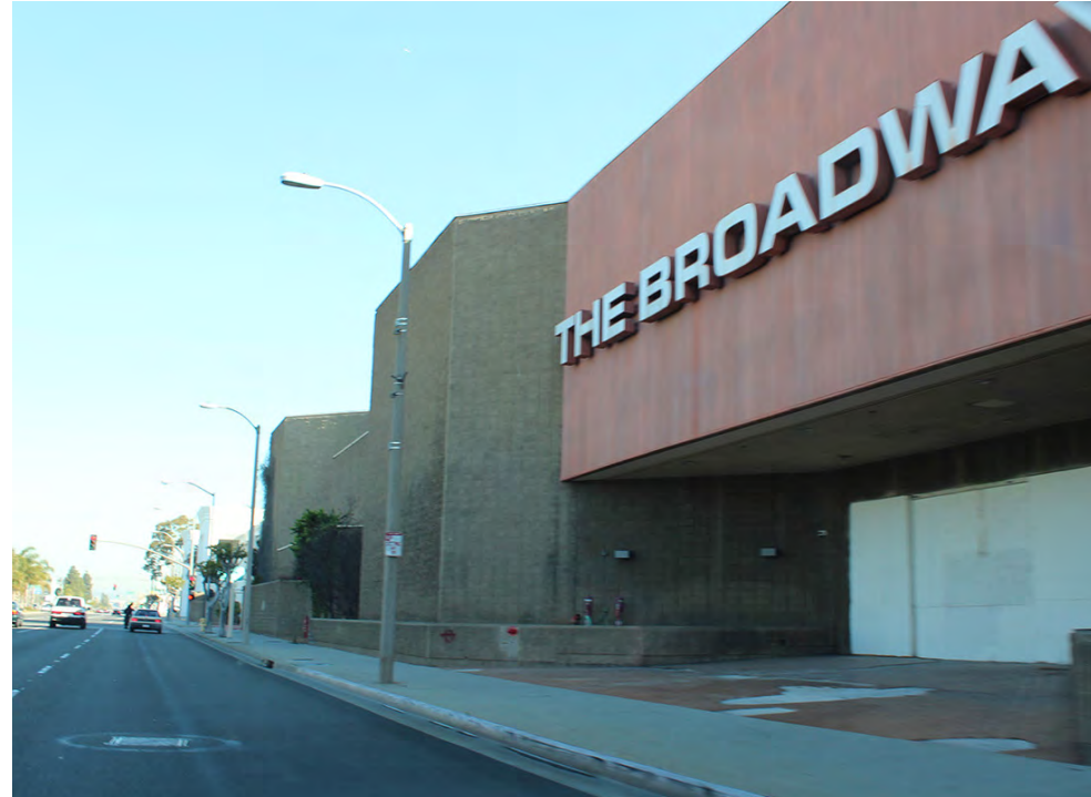
New development should help activate and enliven the street, not deaden it with blank walls and unused, barren spaces
