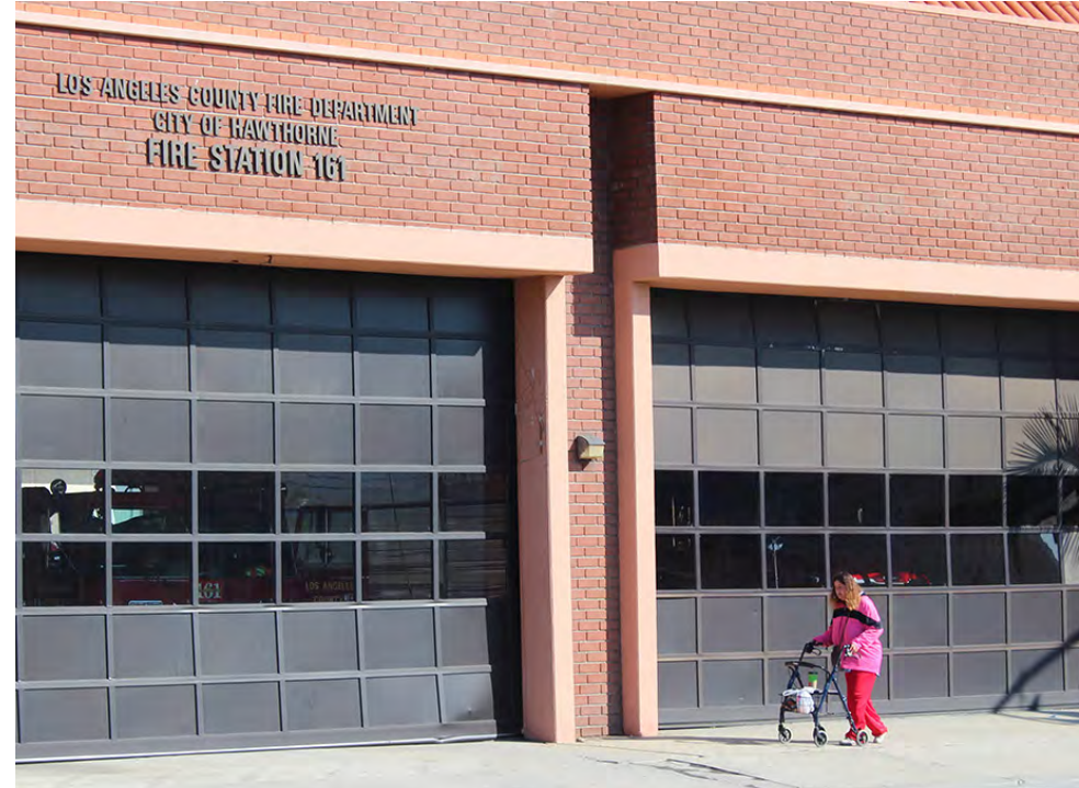
The site currently contains a mix of key public uses, such as a library and fire station, which should be enhanced and expanded upon as new development occurs
