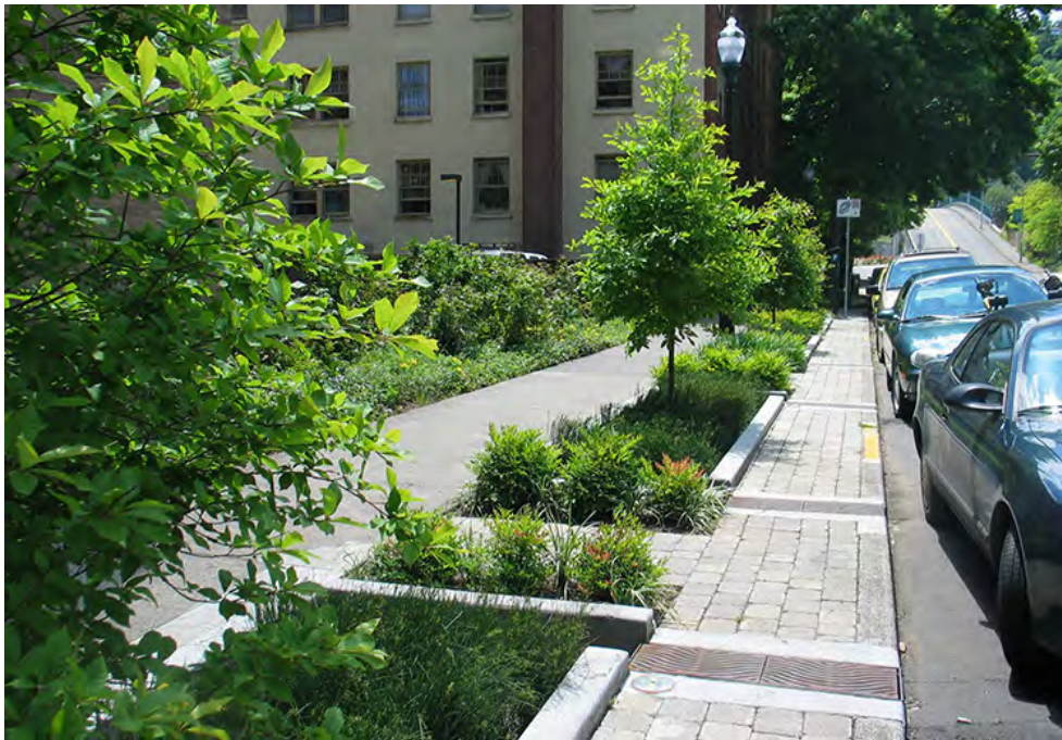
Stormwater planters are a green alternative to traditional drainage techniques, shown here in Portland, Oregon
