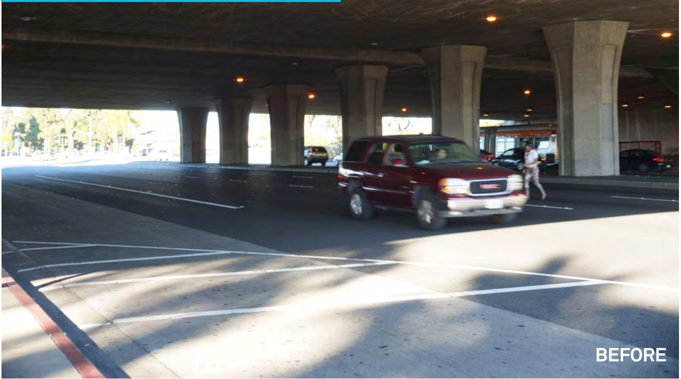
Crenshaw Boulevard and 105 Underpass: Dark, no crosswalk.
