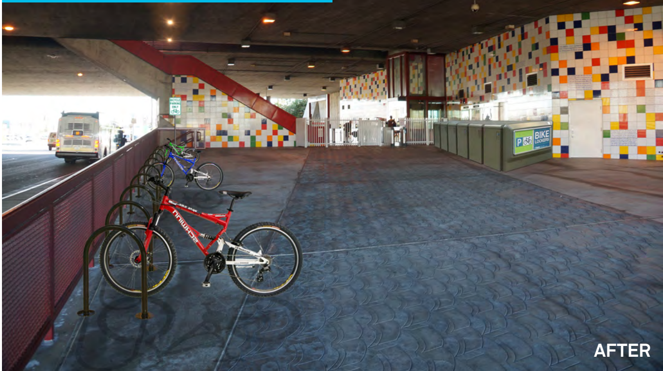
Crenshaw Station: Added lights and bike lockers and racks.
