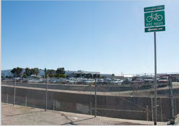
Connectivity – Lack of connections through existing parking lots to Dominguez Channel Trail restricts connections to adjacent businesses.
