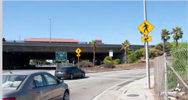
Freeways – The station area contains multiple on/off ramps with no pedestrian signals, double turn lanes, and blind spots at pedestrian crossings.
