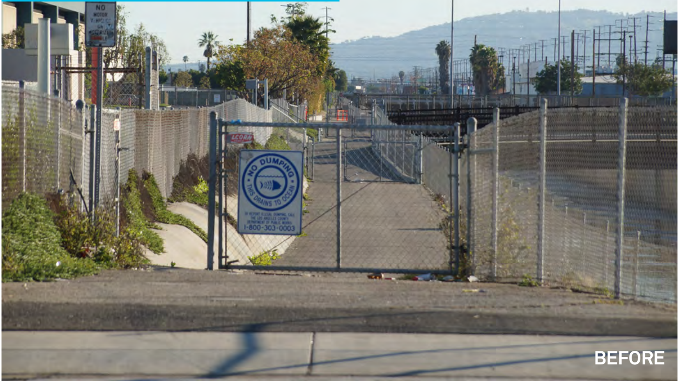
Dominguez Channel Bike Path: In disrepair and uninviting.
