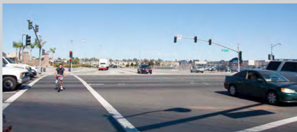
Crosswalks – Crosswalks are very long and contain double-right turn lanes that create blind spots at crossings.
